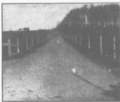
PIECE OF IMPROVED ROAD AT MACDONALD COLLEGE FARM
