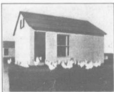
A COLONY POULTRY HOUSE COMPLETED
