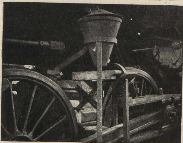
Welding Loco Frame: Ready for Ignition.
