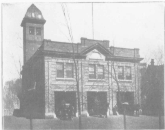
CENTRAL ENGINE HOUSE.
