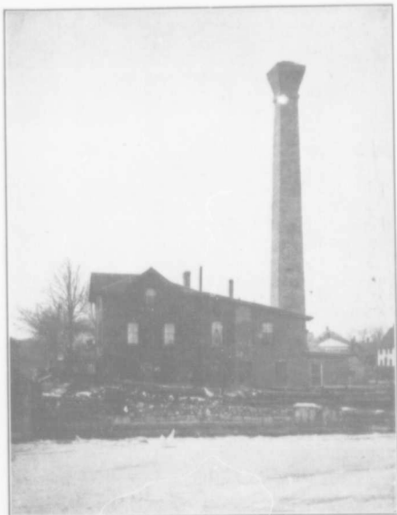
RESERVE AND HIGH PRESSURE PUMP STATION AT RIVER.
