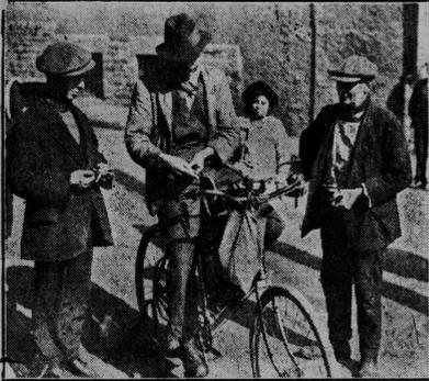
Even the scissors grinder demands a more rapid means of locomotion than pushing the old familiar cart with a couple of grindstones mounted on it. This ingenious scissors grinder mounted a spindle with two carbide wheels on the front of his bicycle frame and supplies the power by means of a small belt from the rear wheel which he cranks while the machine is on a stand. This device enables him to move from one job to another in considerably less time than if he were walking and pushing a cart.
