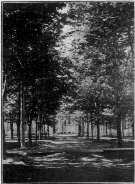
UNION STREET ENTRANCE.
