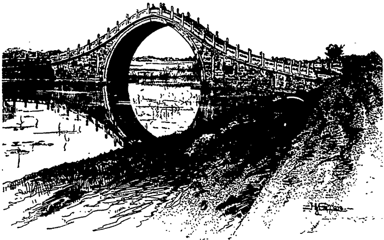
HUNCHBACK BRIDGE, SUMMER PALACE.
