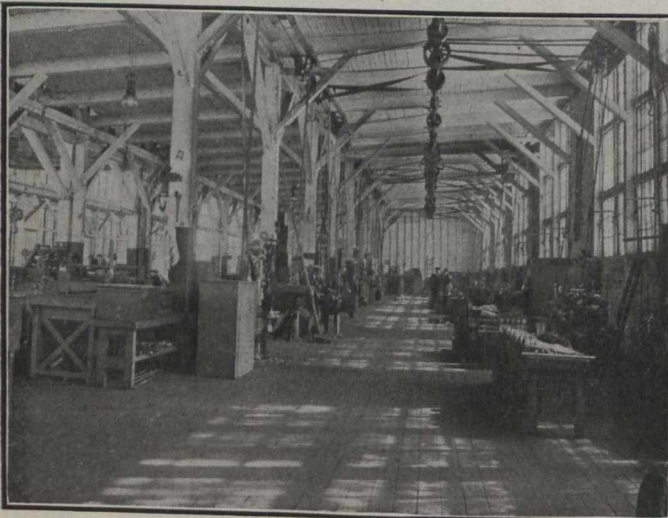
ENGINE DEPARTMENT, UPPER FLOOR—ROBB ENGINEERING COMPANY, AMHERST, N.S.
