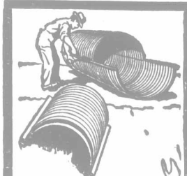
You put Pedlar's Perfect Corrugated Culvert up like this—right at the job
