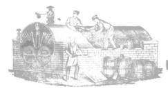
For Coating Boilers' Steam Pipes, and prevent the radiation of heat, save fuel, and increase the power of steam. It will at once Show a Leak; it can not ('atch or Communicate Fire. Used in H. M. Dook yards, Arsensis; also Principal Railway and Dook Co's. Three boilers covered with this composition will do the work of four not covered. May be seen where it has been in use for fifteen years.
