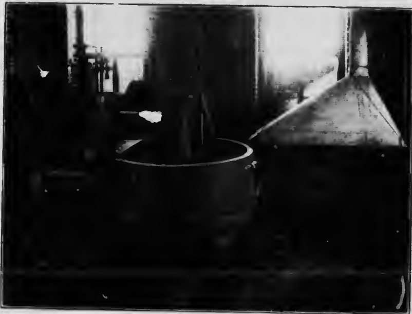
FIG. 6b.—Amalgam Pan, and Settler and Drying Table, Nos. 40, 41 and 48.
