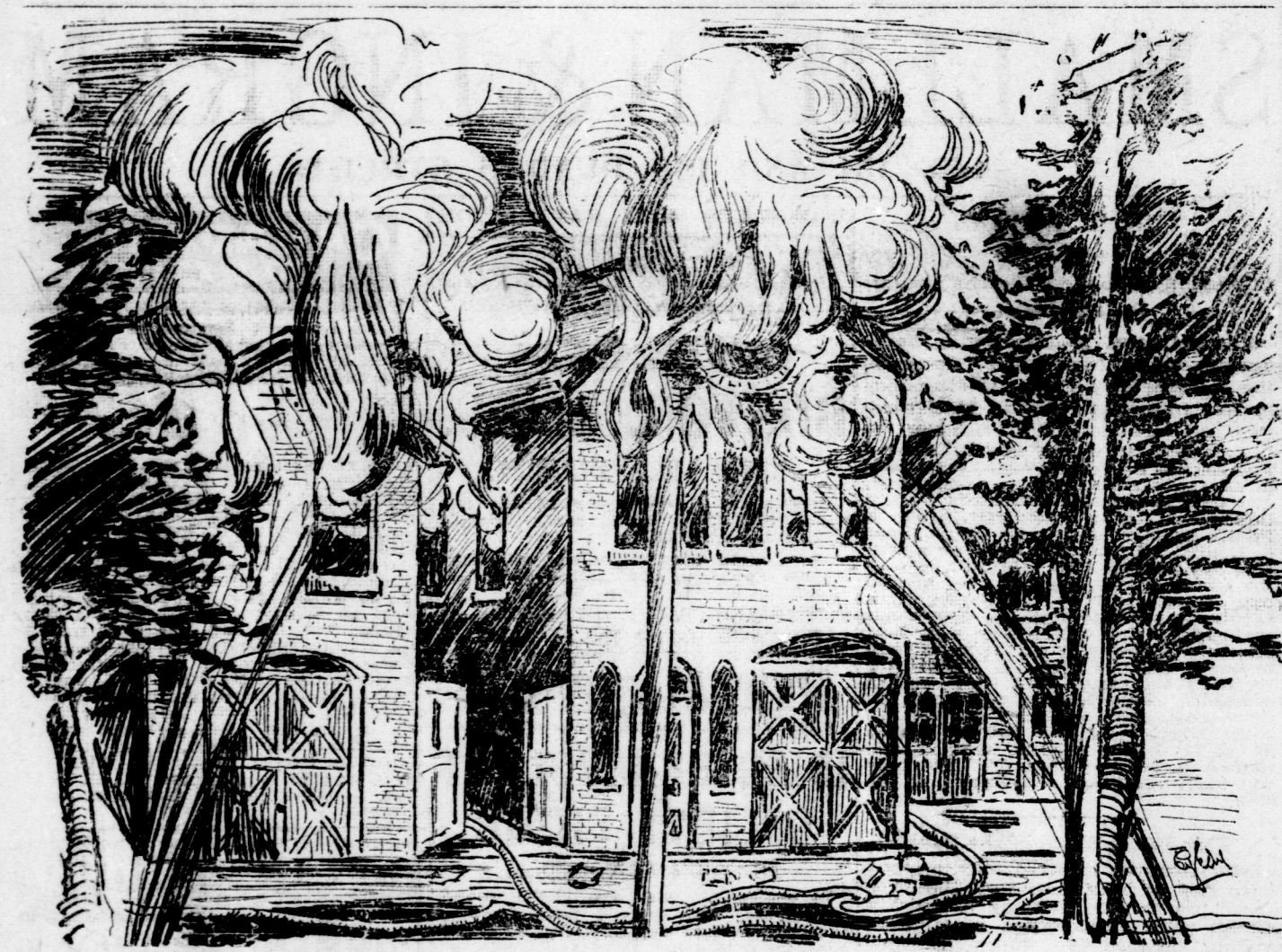
Barns fronting on Dundas Street when the fire was at its worst and other buildings in the neighborhood were in great danger.
