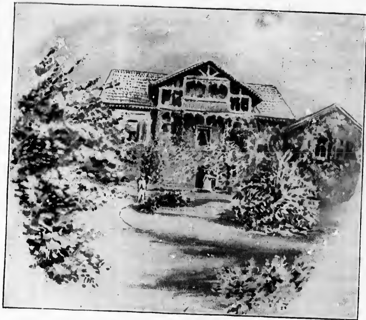
GREAT FRÖEN — THE DWELLING-HOUSE
