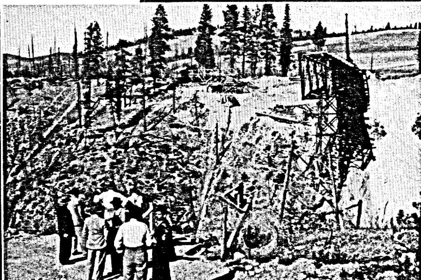
Members of the Highways and Bridge Erection mission from India and Pakistan examine bridge construction in British Columbia.
