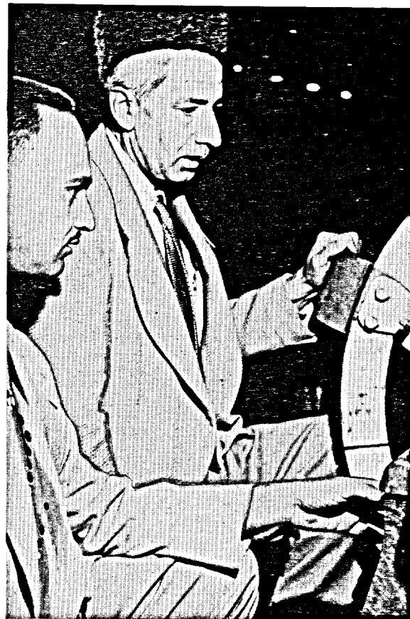
Two members of the Pakistan hydroelectric mission examine a large generator under construction.
