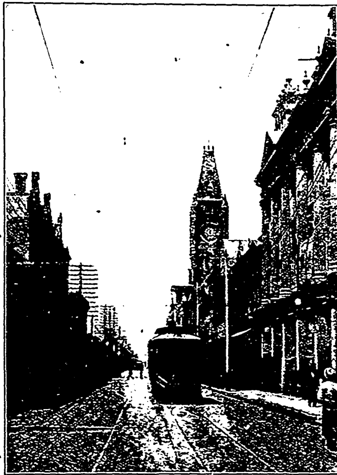
Completed Track, Perth Tramways.
