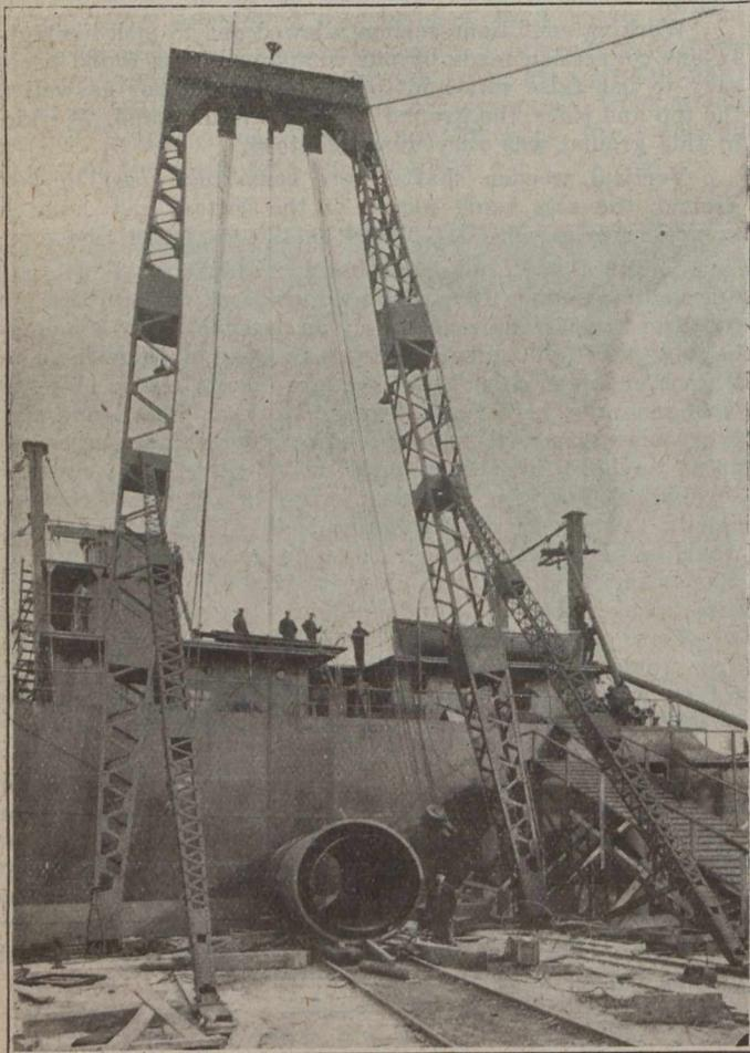
SHEAR-LEGS BUILT FOR DOMINION SHIPBUILDING Co.
