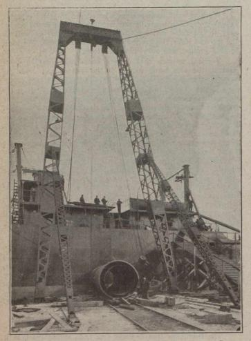
SHEAR-LEGS BUILT FOR DOMINION SHIPBUILDING CO.
