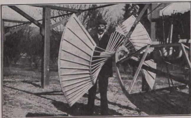
Fig. 2.—View of Fan-shaped Propeller.
