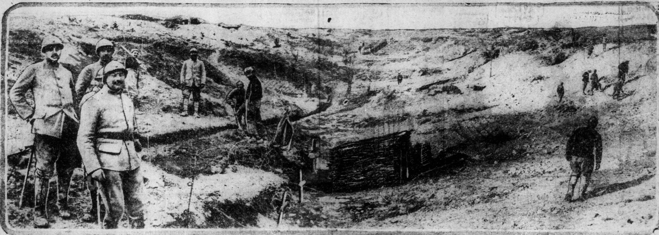
This photograph was taken after the present German offensive northeast of Verdun was commenced, and gives an idea of the character of the terrain. French soldiers are shown repairing the trenches and underground shelters after a heavy bombardment. Note the crosses marking freshly-made graves.—(Exclusive Courier Pictorial Service, in conjunction with the London Daily Mirror.)
