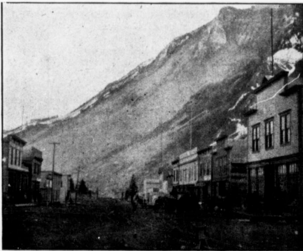
View of the slide from Main Street.
