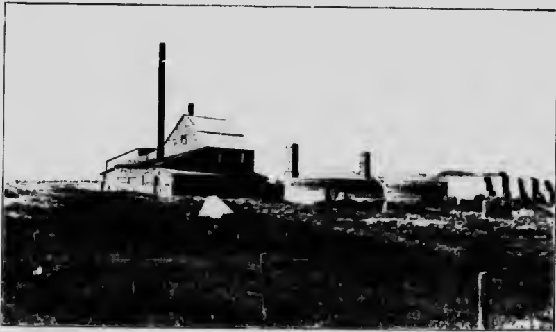
Plant of the Weyburn Brick Company, Weyburn, Sask.
