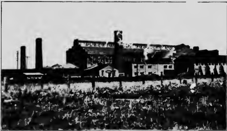
Sewerpipe plant of the Alberta Clay Products Company, Medicine Hat, Alberta.
