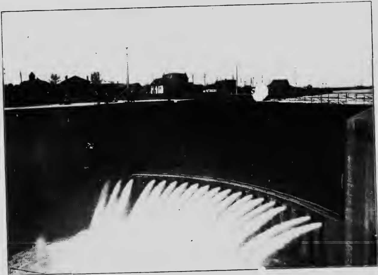
Filling the Under Channels of Poe Lock Preparatory to Opening for Navigation.
