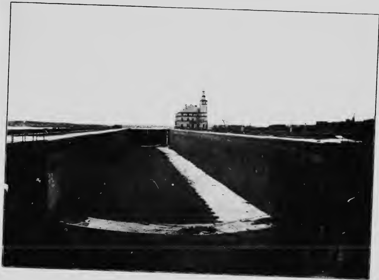
General View of Poe Lock Before Being Filled for Navigation.
