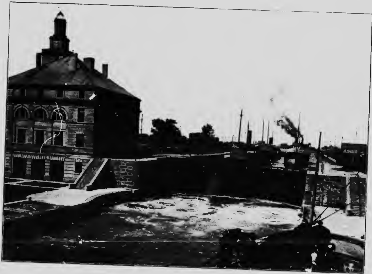
Poe Locks General View Looking West.
