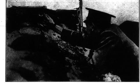
Dutch soldier firing rifle, using the "Eradus" periscope. This device was designed by J. H. Eradus, a Dutch inventor, and is named in his honor. It is attached to the butt of the rifle and enables the soldier in the trench to aim and fire accurately without danger of death from the enemy's bullets. It is in use in the Dutch army and should revolutionize sniping along the battlefronts.
