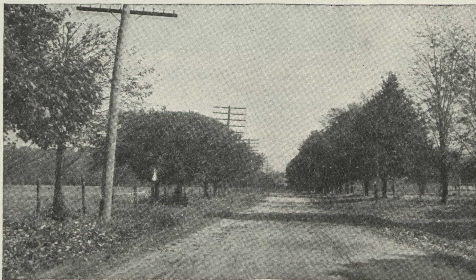
Tree-Planting Transforms Country Roads
