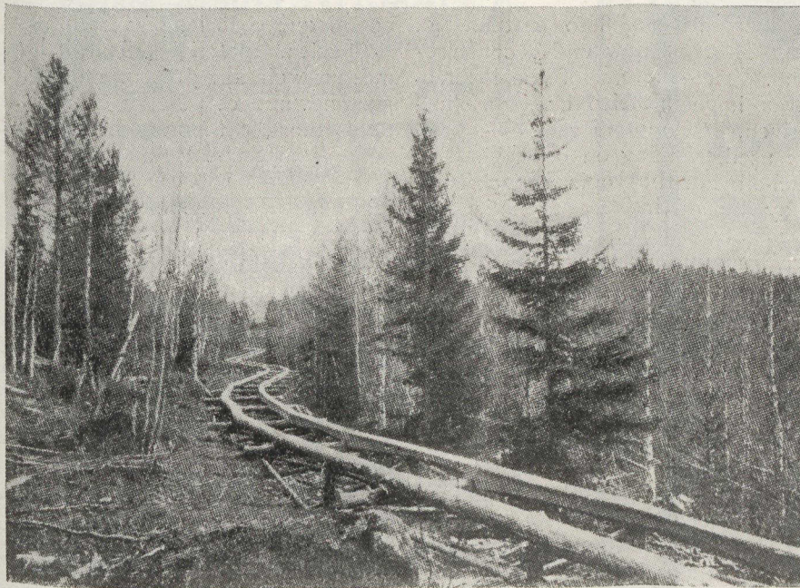
A Swedish wooden railroad made possible by the invention of a peculiar car wheel, not flanged, which obviates wear and operates with remarkable safety. The wheels are rubber-tired. (See accompanying article.)
