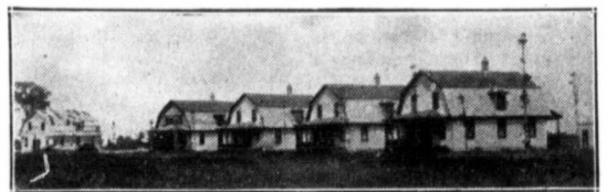
These substantial Workingmen's Houses are built by the Hiram Walker Co., Walkerville, Ont., using Stucco laid on a foundation of
