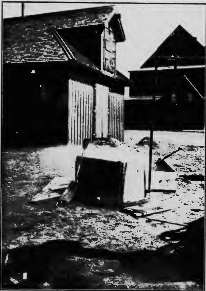
Figure IV. Sterilization of soils. (Steam is forced, for 30 minutes, into the closed box which is filled with soil to be treated.)
