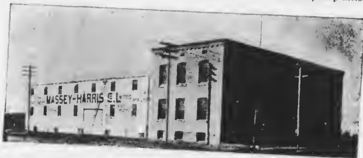
One of our Fifty Implement Firms,—The Massey-Harris Co.'s Offices, showing portion of warehouses to rear.
