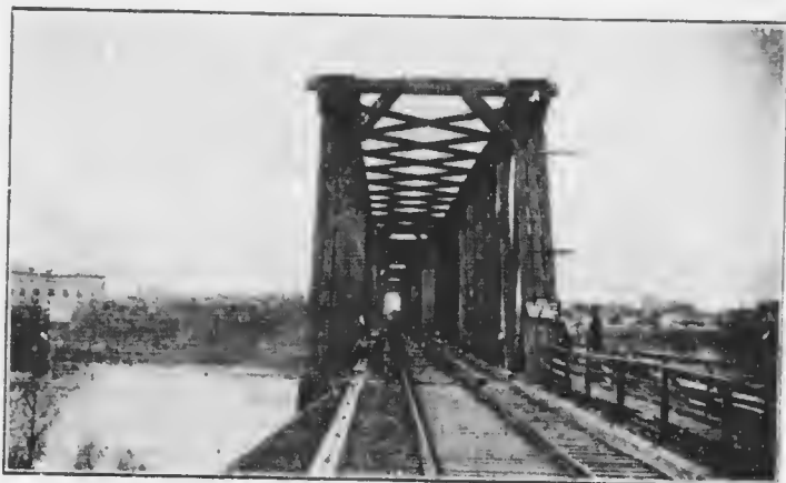
Canadian Northern Railway Company's Bridge.—one more of our four
