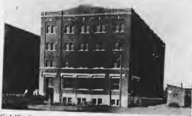
The Codville Co.'s New Warehouse their old premises having become entirely inadequate for the handling of vastly increasing business.
