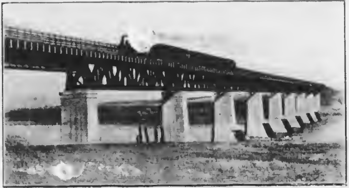
Canadian Pacific Railway Company's Bridge, length 1,300 feet. One of Saskatoon's four bridges. A fifth now in prospect.
