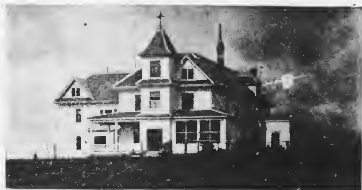
Saint Paul's Hospital, A Splendid New building in process of erection.
