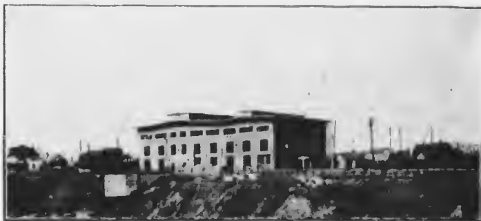
New City Power House the highly modern equipment of which places it in a lone class.
