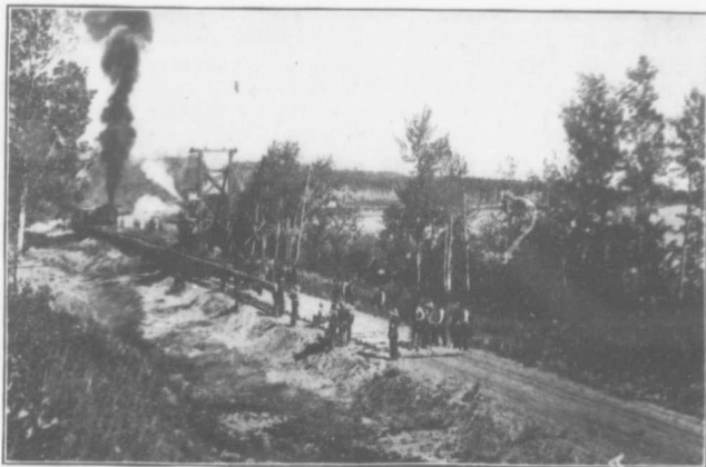
BUILDING THE GRAND TRUNK PACIFIC WEST OF EDMONTON
