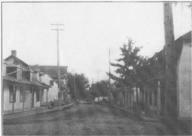
A STREET SCENE IN A QUEBEC VILLAGE NEAR MONTREAL
