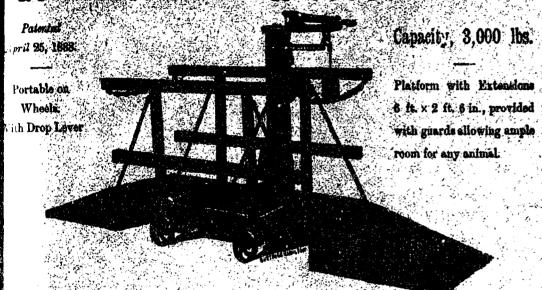
onstructed that Extensions and Guards can be imcompled when desired, and Scale used without them, his Scale was first introduced in 1888. We sold more Scales of this description in 1891 than we did in the three former years put together, showing its increasing popularity.
