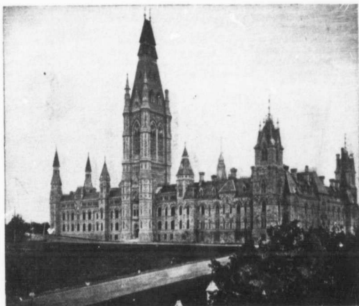
WESTERN DEPARTMENTAL BLOCK.
