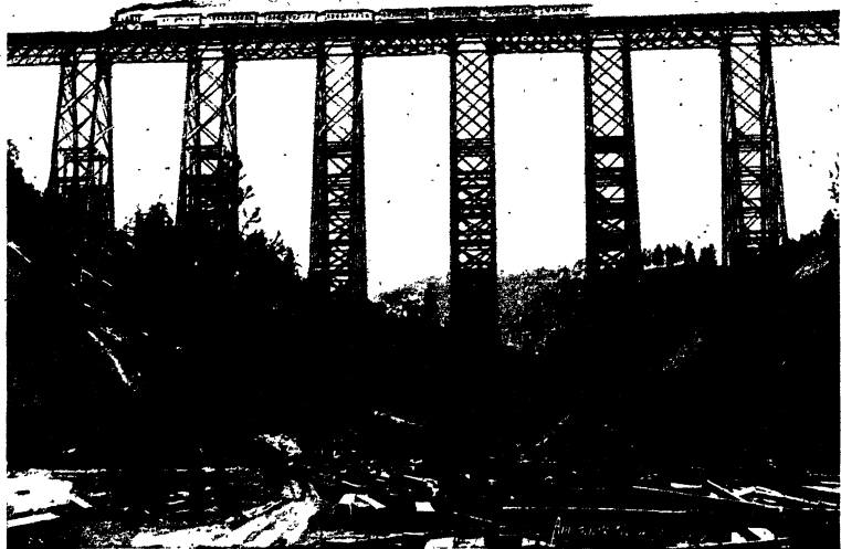
MARENT TRESTLE, 226 FEET HIGH.
