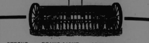
STRONG DRAWS LIGHT SEEDS ACCURATELY. The Frame of a Drill is its Foundation. It must carry the weight of the hopper above and the strain of the pressure below without springing or sagging, in order to make light draft. It must also keep the working parts in proper alignment to ensure accurate seeding. Note how completely these objects have been attained in the
