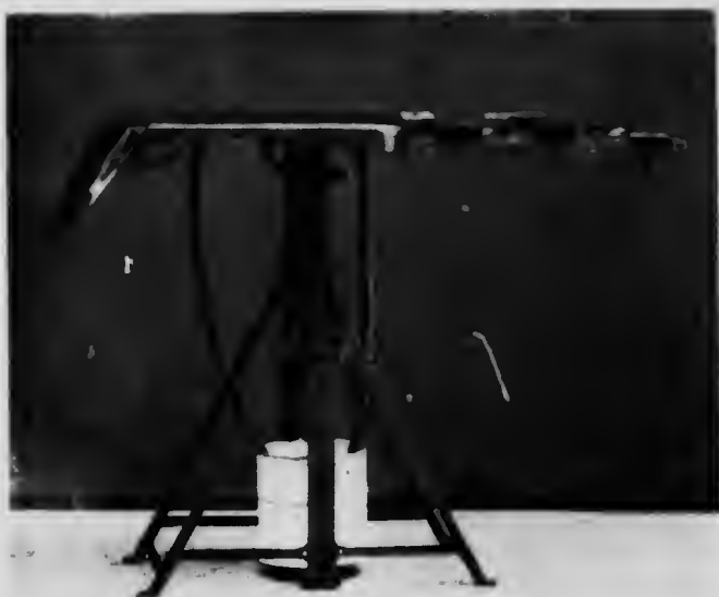
FIG. 17. AUTHOR'S TRANSPORTABLE OPERATION-TABLE. Rose's position; leg-supports adjusted horizontally.
