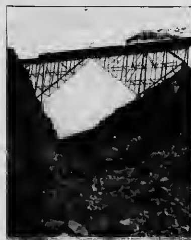
Steel Cantilever Bridge near the Summit of White Pass
