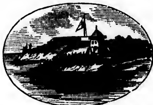
FORT HENRY—MARTELLO TOWER. CEDAR ISLAND.
