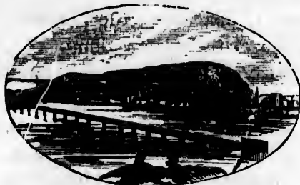
MONTREAL, AND VICTORIA BRIDGE.
