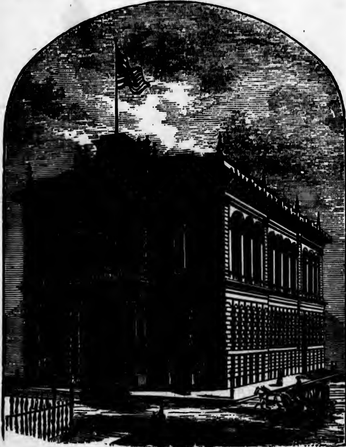
CHAMBER OF COMMERCE AND BOARD OF TRADE BUILDING, CHICAGO.
