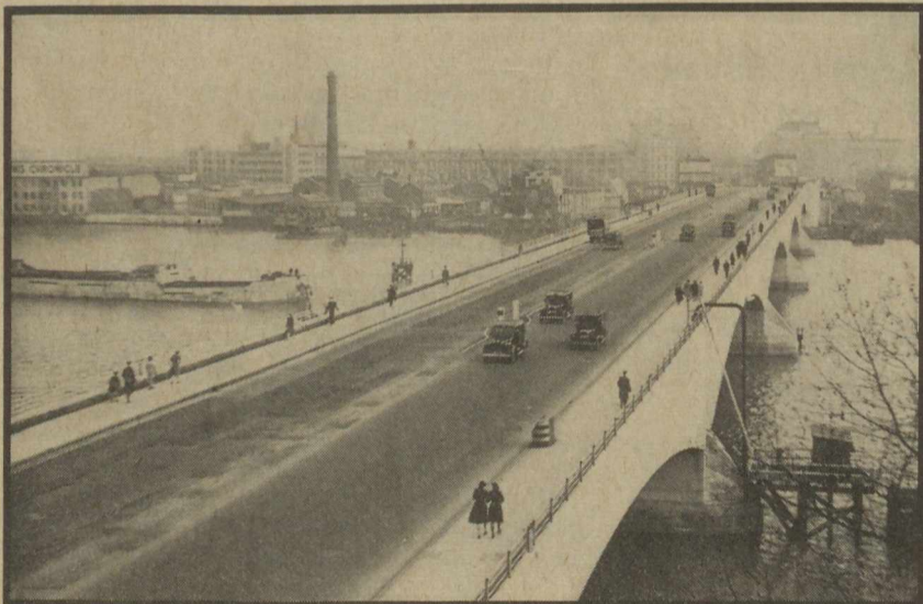
Britain's courageous perseverance in the face of almost continuous bombing is exemplified in the construction of the new Waterloo Bridge, spanning the Thames in London. Begun before the war, work on it continued all through the Blitz, and although not completed, it was opened without ceremony to two-lane motor traffic in 1942. More recently, as this photograph shows, it was thrown open to six lanes of traffic.
