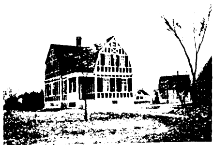
One of a group of cottages covered roof and sides with our roofing.
