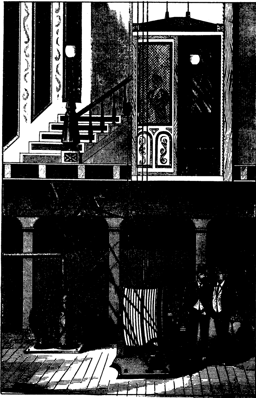
ELEVATOR WORKED BY THE SHERRILL ROPER ENGINE.
