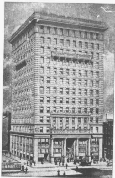
STEPHEN GIRARD BUILDING, PHILADELPHIA. HEADQUARTERS OF THE SUN LIFE OF CANADA, FOR PENNSYLVANIA.
