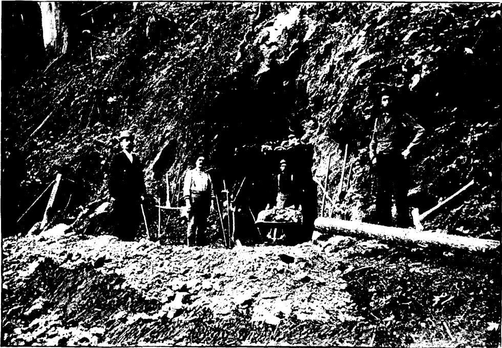
ORE DUMP—GOLD EAGLE MINE.
