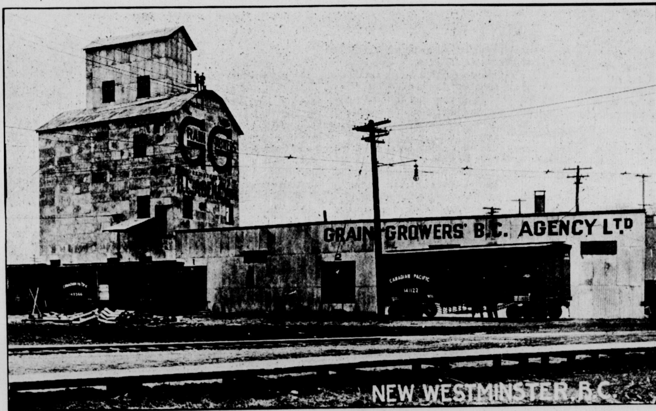
The above is the new elevator, warehouse and feed mill, purchased by The Grain Growers' Grain Company at New Westminster, B.C., in October last. It is one of the most complete plants of its kind in Western Canada, and is doing a big and growing business with the poultry and dairymen of the Fraser Valley and Vancouver Island. The mill has a grinding capacity of 100 tons per day, and will make a splendid outlet for oats and barley and the lower grades of wheat, for Alberta farmers who can ship to it via the C.P.R. This plant is being operated under the name of The Grain Growers' B. C. Agency Ltd.
