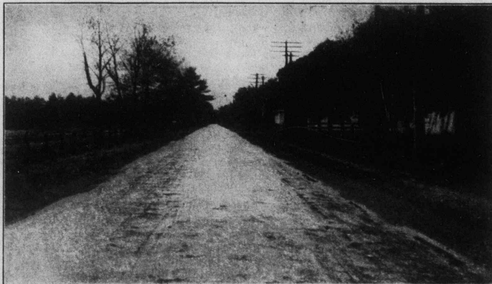
A Bituminous Surface Treatment, using an oil carrying 70 per cent. of asphalt.
