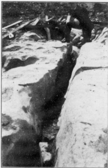
View of deep crevice opened in bedrock by the river currents at Electrical Development Company's Forebay.
