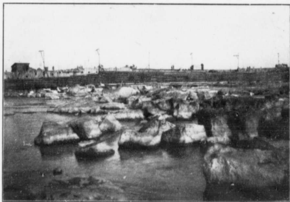
View of Bed of River at Electrical Development Company's Forebay when water was drained off. The joints in the bed rock opened by solution of the limestone, leaving separated masses still in place.
