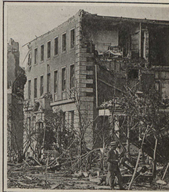
A Bedroom Suddenly Exposed to View.
