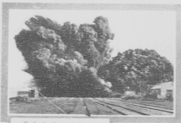
The last big blast on the Yosemite Jan. 21, 1914
