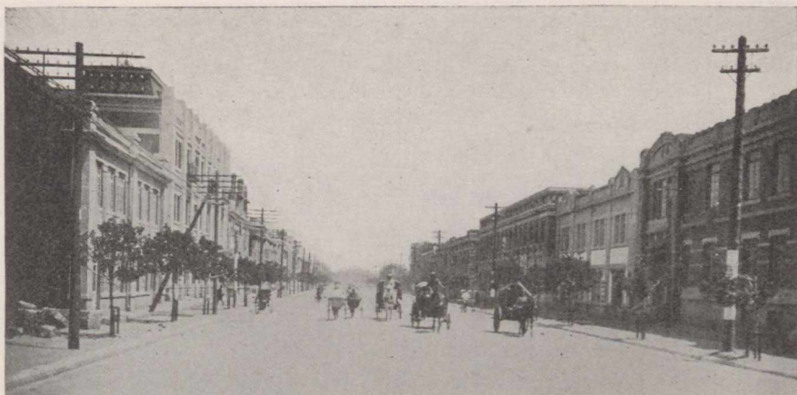
Fig. 11 illustrates a street in the Japanese portion of the city of Mukden
