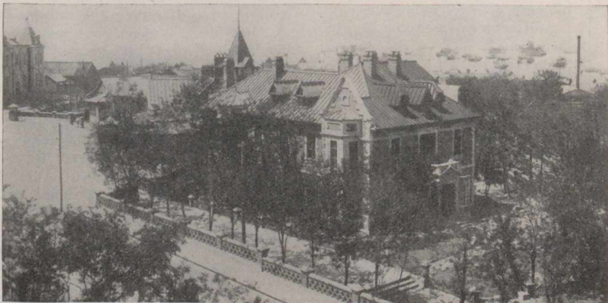
Fig. 4 shows a training school for railroad employees
