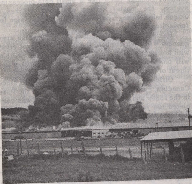
St. Joseph de Beauce factory goes up in smoke.
