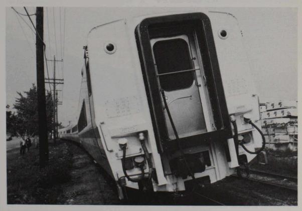
The unique banking system of Bombardier's LRC trains allows them to negotiate sharp curves at high speed.
