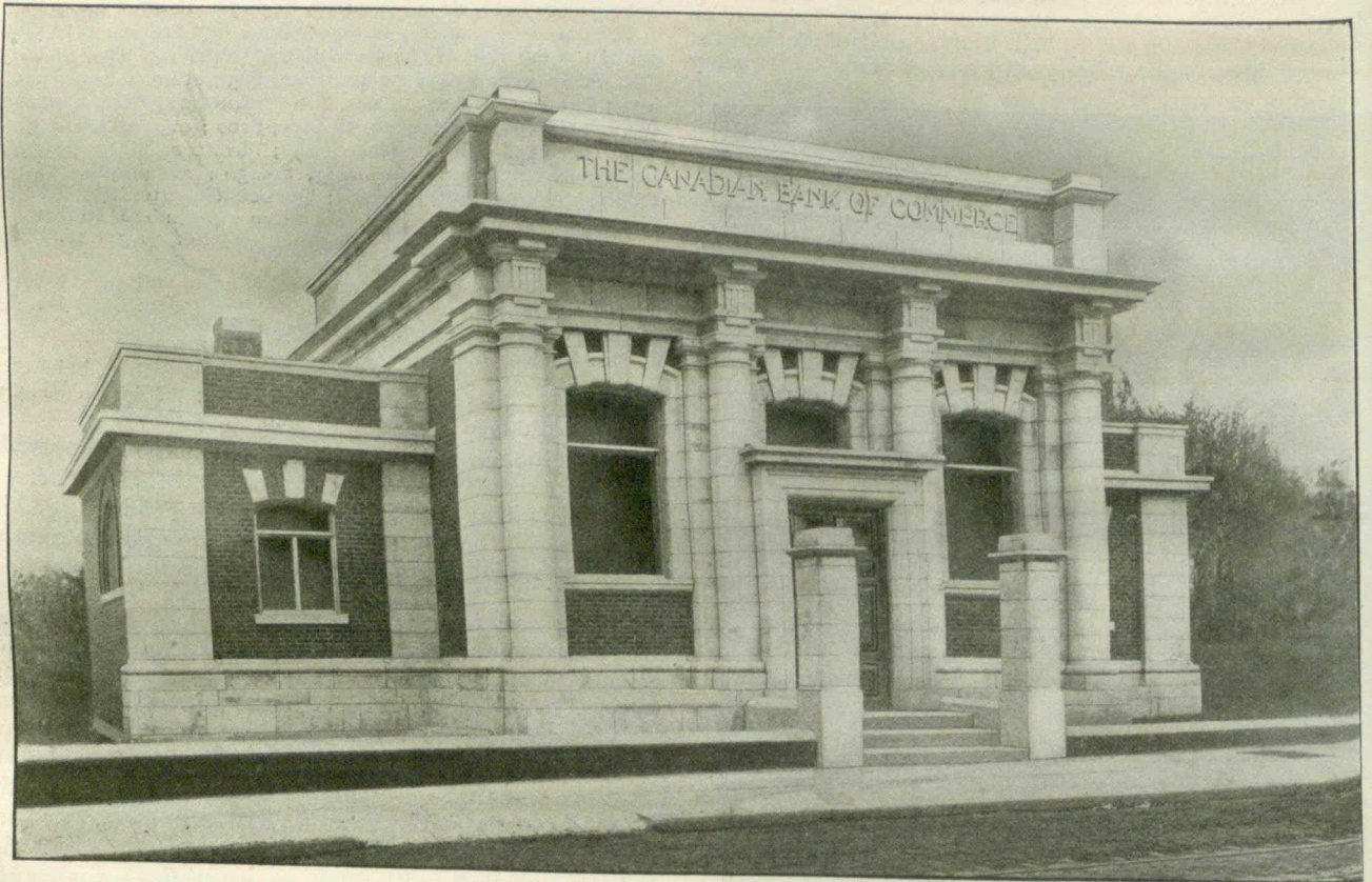
PARKDALE BRANCH CANADIAN BANK OF COMMERCE, TORONTO.—DARLING & PEARSON, ARCHITECTS. The building is constructed of brick with Roman Stone trimmings, giving a very satisfactory appearance.
