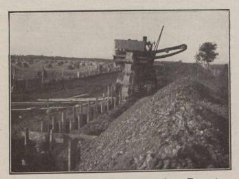
Fig. 4—Excavating 20-ft. Trench from Town to Disposal Works.
