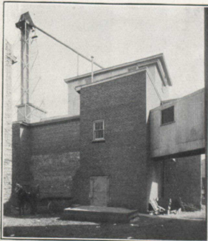
215-221 Eighth Street East Long Distance Telephone 183 Local Orders and Shipping Room 172
